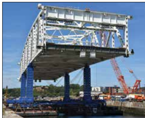
One JS-250 Jack-Up Unit with Barrel Sets installed
