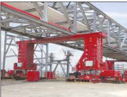
▼ Lifting an oil and gas pipe module
